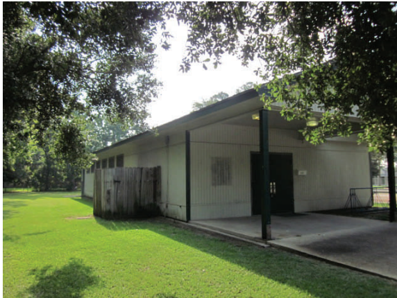
Recreation Center Prior to Improvements
