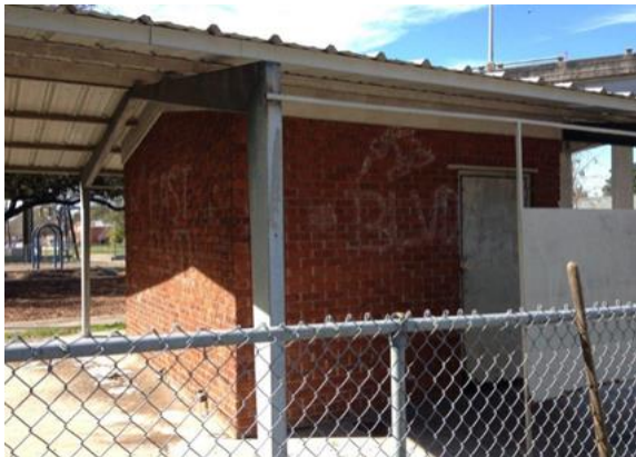
Restroom Building Before Demolition
