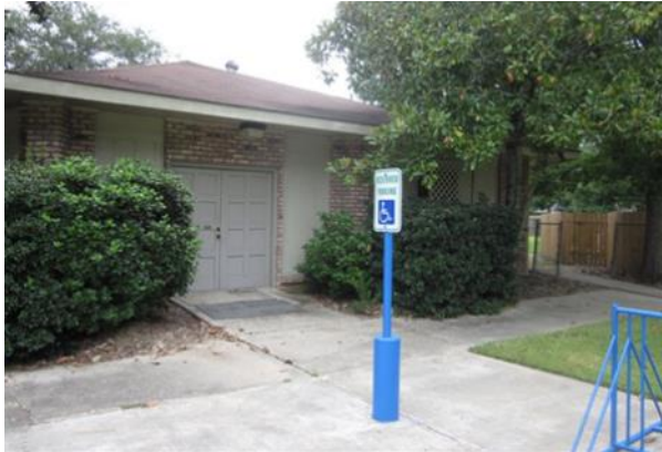
Recreation Center Prior to Improvements
