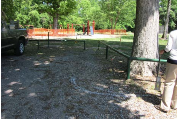
Parking Area before Improvements
