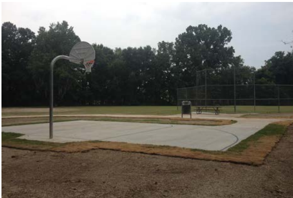
New Half Basketball Court
