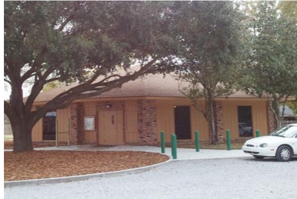
Newly Painted Center & Improved Parking Area
