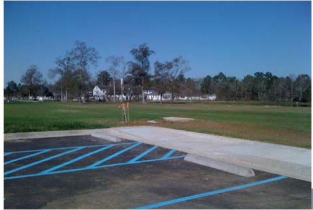
New Asphalt Parking
