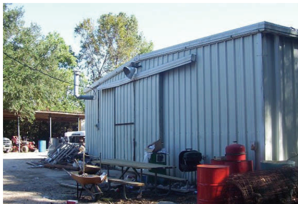
Old Maintenance Facility
