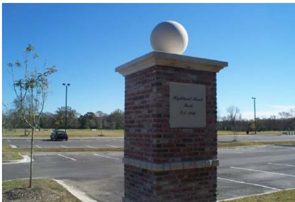
New Pilaster & Parking Lot
