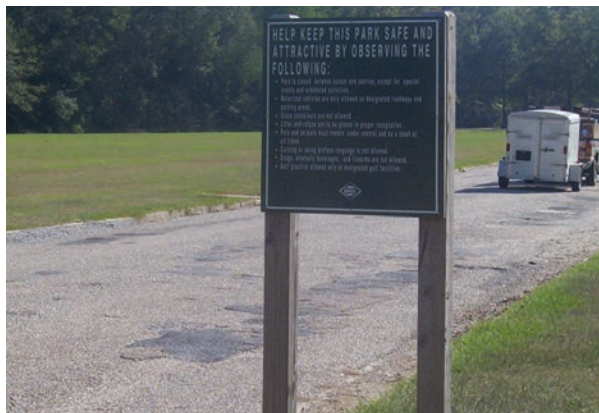
Park Road Prior to Improvements
