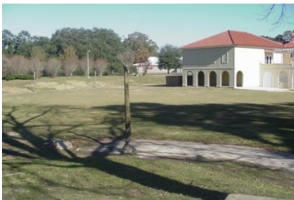
Back of Art Gallery Prior to Improvements
