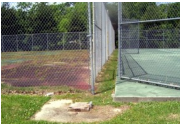
Tennis Courts Prior to Improvements
