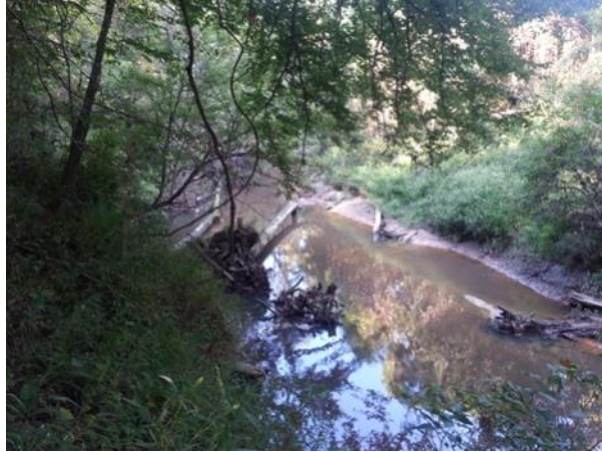
View of Sandy Creek
