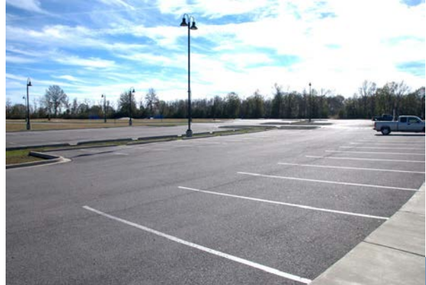
Paved Parking Lot with Lighting
