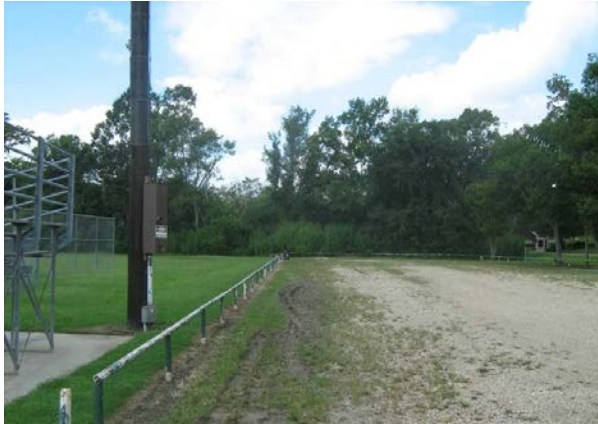
Gravel Parking Lots Near Ball Fields Before
