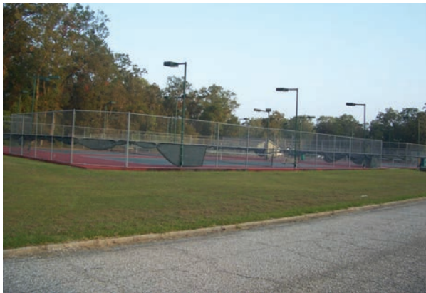
Tennis Courts Prior to Improvements
