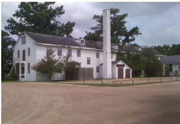
Former Administration Building
