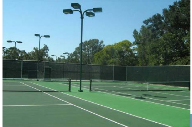
Tennis Courts After Renovations
