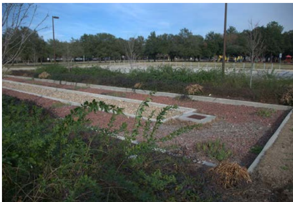
New Paved Parking With Lights & Rain Garden
