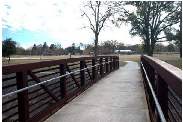
New Pedestrian Bridge
