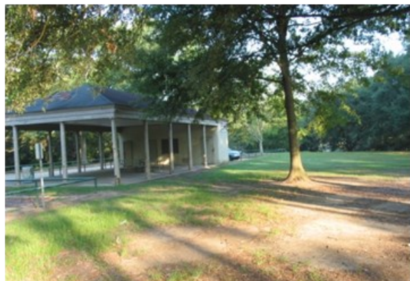
Picnic Hill Prior to Improvements
