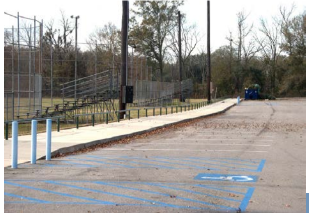
New Paved Parking
