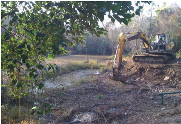
Site Construction For New Pavilion
