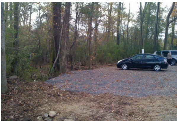
Parking & Site Drainage Improvements
