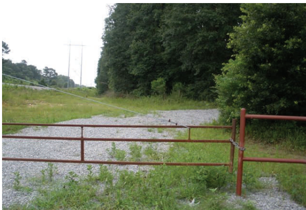
Site Before New Trailhead Construction
