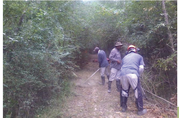
CIP Crew Clearing Trails
