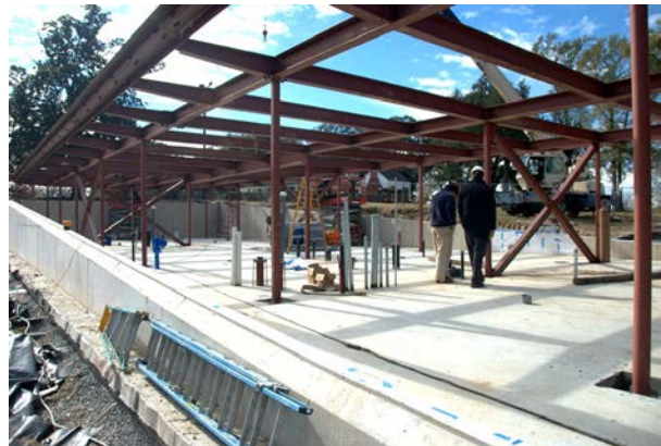
Visitor Center Under Construction
