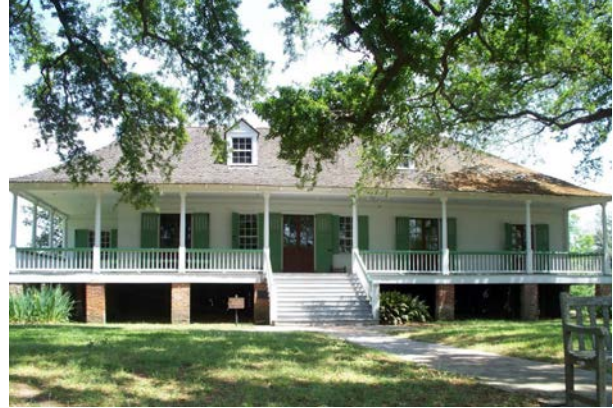
Plantation Home After Renovations
