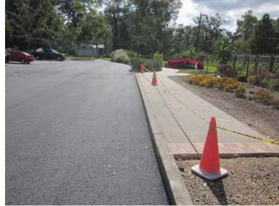
Repaved Parking Lot
