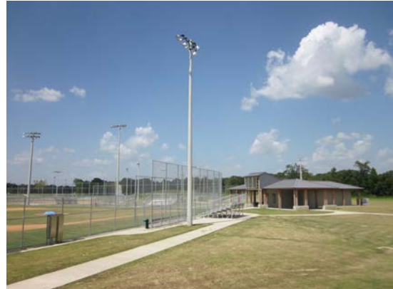
View Of Concession Building
