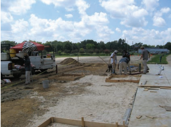
ADA Parking— Under Construction
