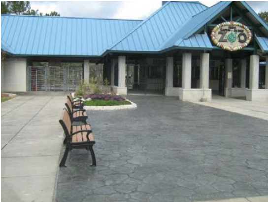
Refurbished Entry Plaza
