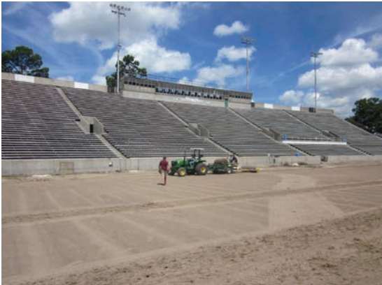
Football Field—During Construction
