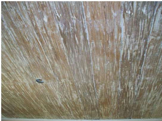
Interior Before Painting
