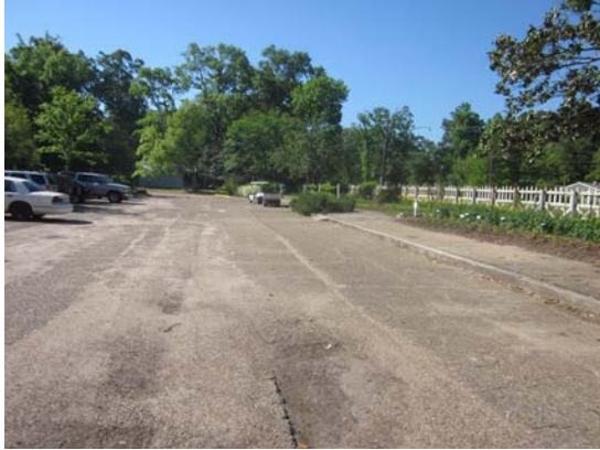
Parking Lot Prior to Improvements
