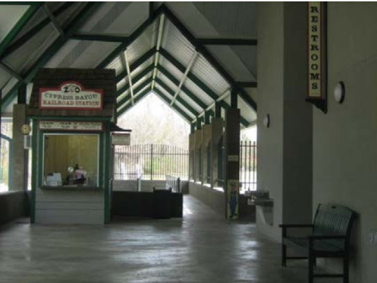
Refurbished Cypress Bayou Railroad Station
