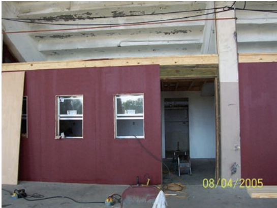
Concession Stand— During Construction
