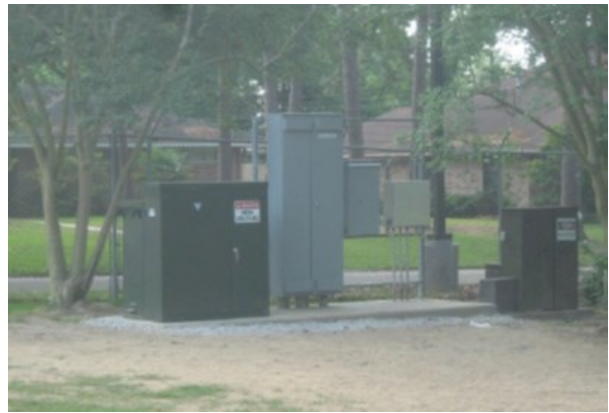
New Electrical infrastructure
