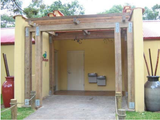
New Restroom Facilities
