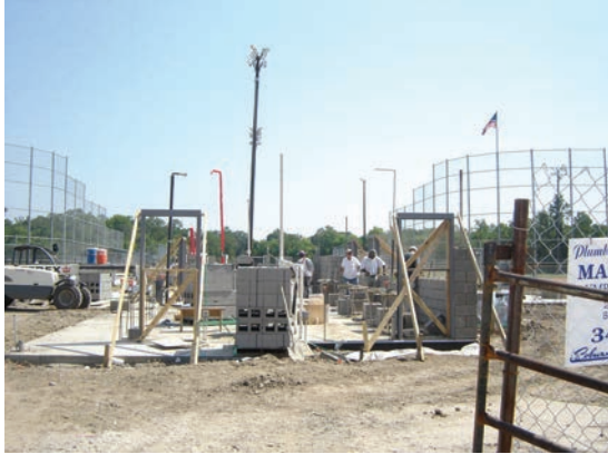
Concession Building Construction
