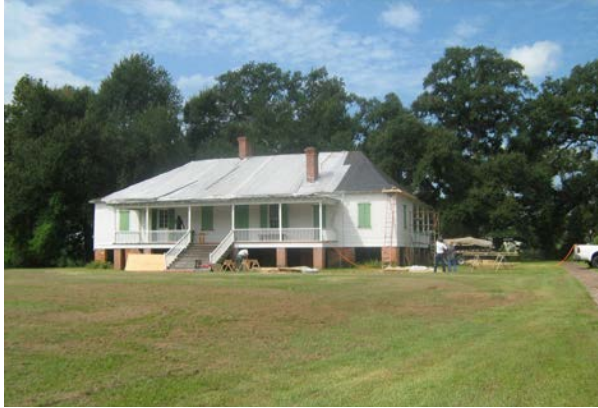
Plantation Home During Renovations
