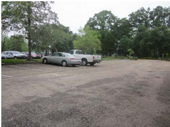
Parking Lot Prior to Improvements
