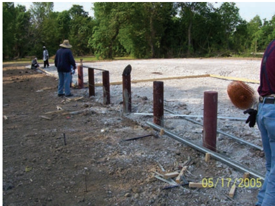
Neighborhood Park—During Construction
