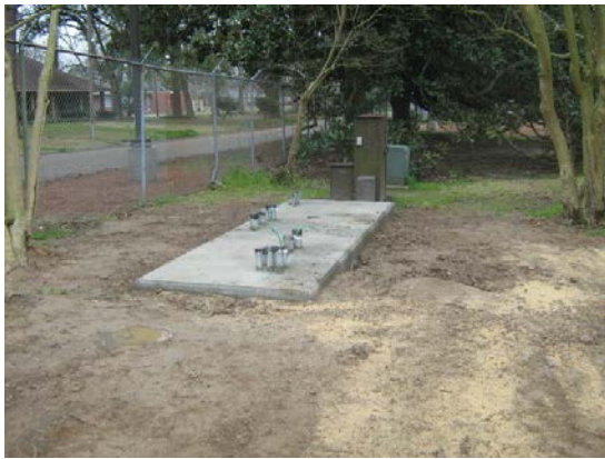
Electrical Infrastructure Installation
